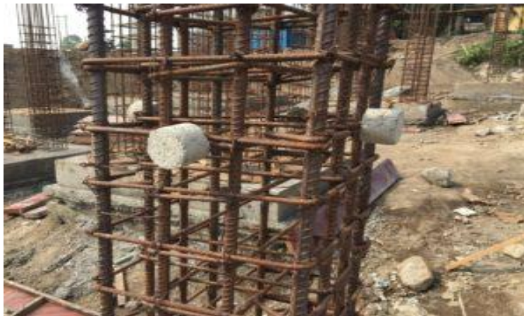
Fig.1 Cover block at site.
