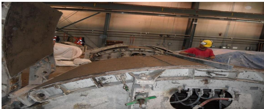
Figure.2 – Demolding process of PCTL segment at fabrication plant
