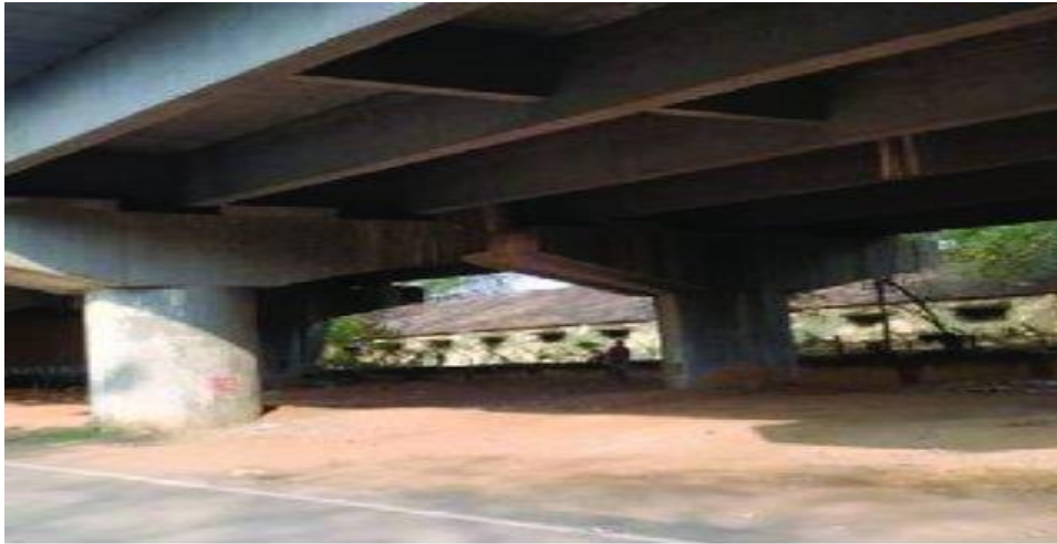
Fig.1 Bridge actual photograph
