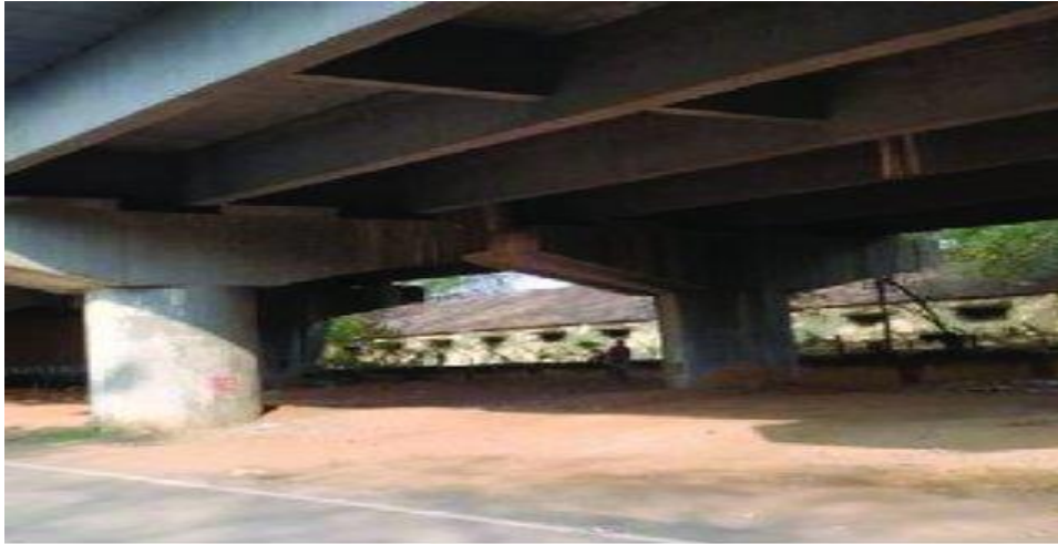
Fig.1 Bridge actual photograph
