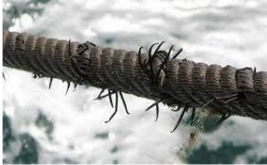
Fig 1 Wire rope failure
